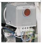
Control box fitted with an ignition transformer
