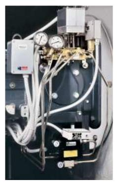
Example of the MB 4 LE burner hydraulic circuit
