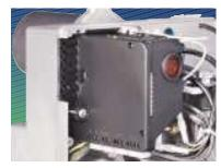
Appliance fitted with an ignition transformer
