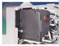
Appliance fitted with an ignition transformer
