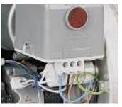
Control box fitted with an ignition transformer
