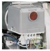
Control box fitted with an ignition transformer
