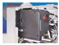
Appliance fitted with an ignition transformer
