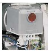
Control box fitted with an ignition transformer
