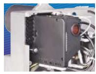
Appliance fitted with an ignition transformer
