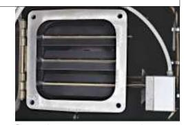
Example of the servomotor and dampers for air setting
